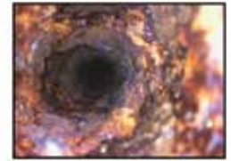
Corrosion Products Rust/Calcium Carbonate
